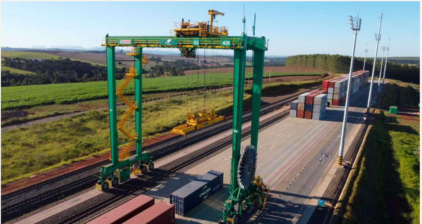
Klabin's Container Terminal (KBT), located next to the Puma Unit in Ortigueira (PR), centralizes the export volumes from the Puma and Monte Alegre plants, which are transported to the Port of Paranaguá.
